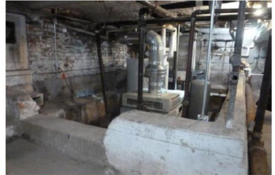
Dry component floodproofing is often an effective solution for equipment that cannot be elevated or relocated out of basements.
