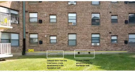
Figure 5- Typical penetrations along the foundation walls
